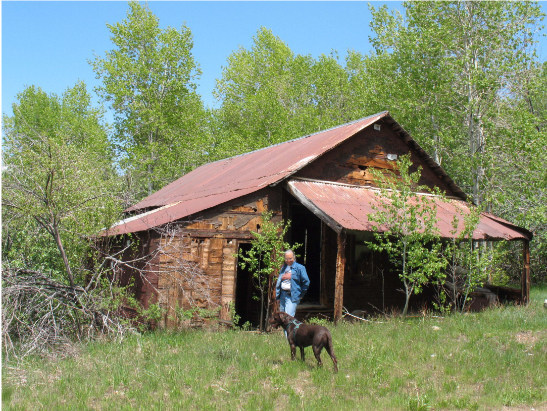
Photo 4.10. An abandoned structure in the canyon below Blue Jacket mine.
